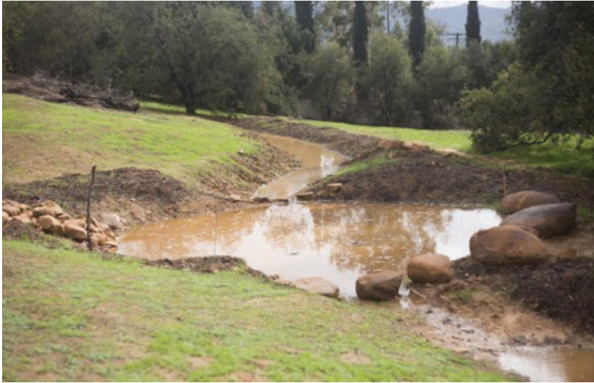
Swales and an infiltration pool holding water that previously deposited silt on highway 33 and wasted copious amount of water. Designed and installed by Connor Jones.
